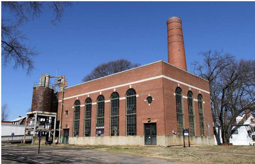
Fig. 5. UMW Heating Plant at College Avenue and Powhatan Street, Fredericksburg, VA. Heating Plant is fueled by natural gas and produces steam used for heating air and water in buildings across campus.
